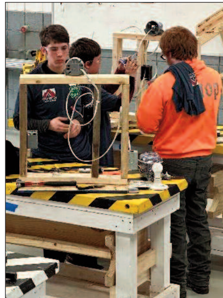
Youth were taught the basics of electricity and how to wire an electrical socket.
